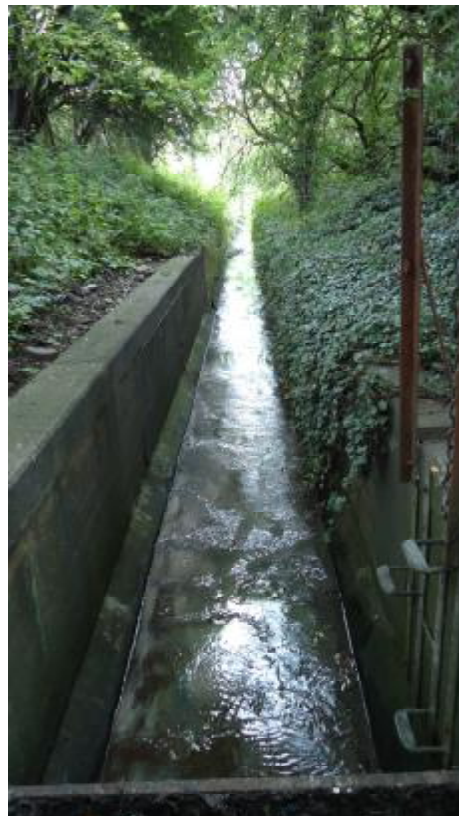
Looking down stream—The Wharf Brook
