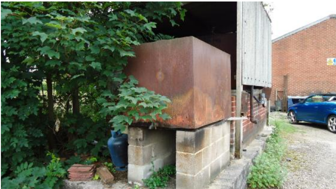
ASTs adjacent to the vehicle repair works
